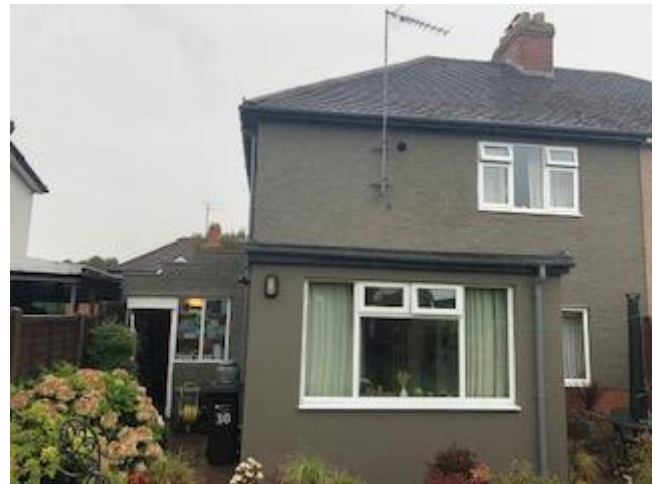
Site photo of rear of No. 30 (adjoining dwelling)
